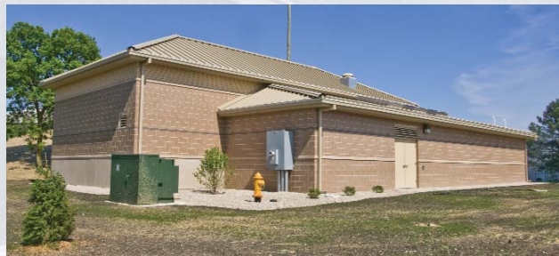
Well 30 - Palo Verde Drive
