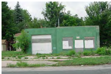
Abandoned commercial buildings provide opportunities for redevelopment.
