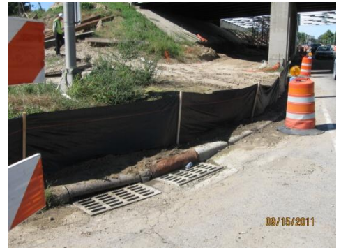
Back of curb silt fence in place to keep sediment from entering the street and storm inlets.
