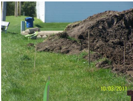
No perimeter silt fence installed allowing sediment to leave site.
