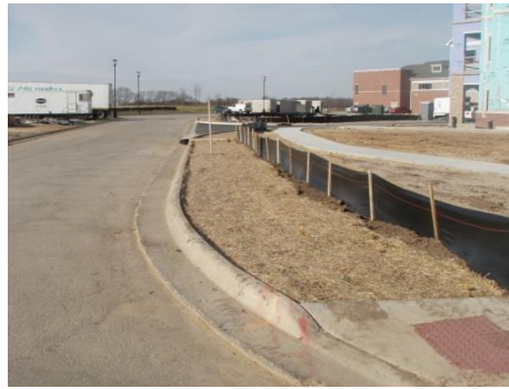
Back of curb silt fence in place to keep sediment from entering the street and storm inlets.
