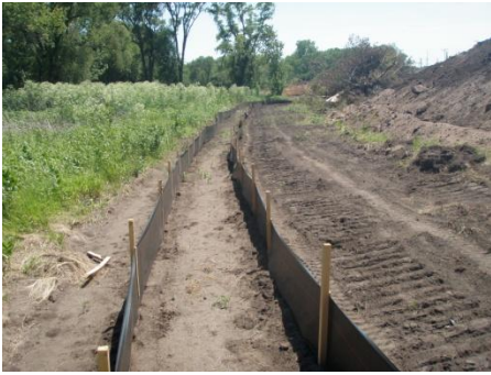
Properly maintained and installed perimeter silt fence
