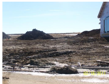
No perimeter silt fence installed allowing sediment to leave site.
