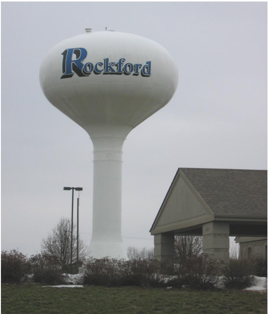
The elevated tank on W. Riverside Blvd was built in 1985 and holds 1,500,000 gallons. Photograph provided by Thomas Powers
